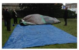
2 Remove tower section from its bag, carefully unroll it and spread it out.
